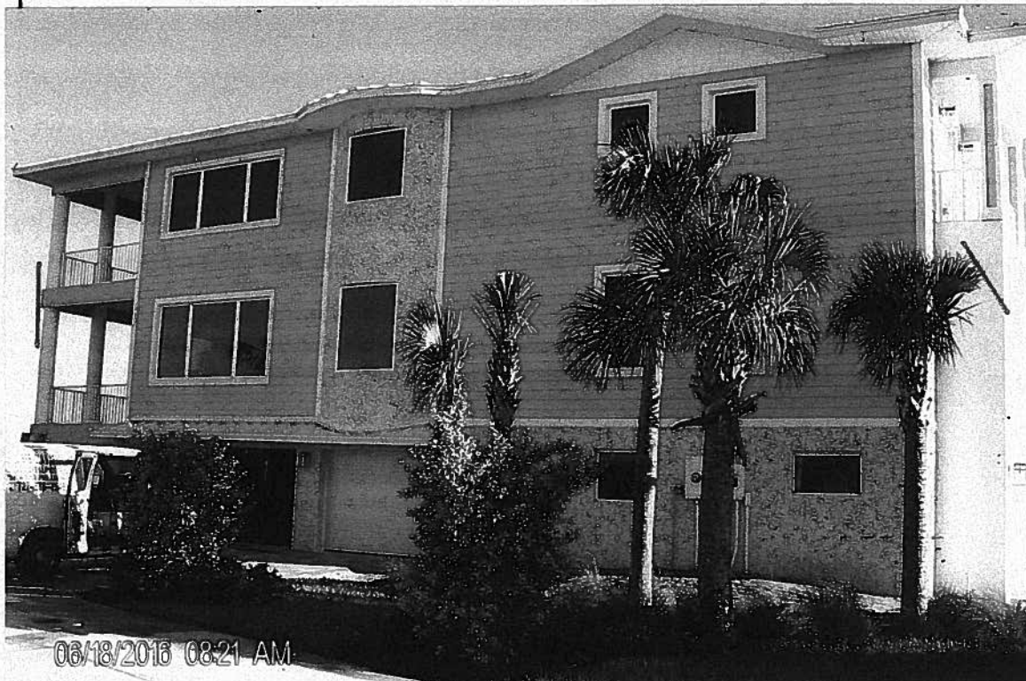
SOUTH SIDE OF BUILDING
